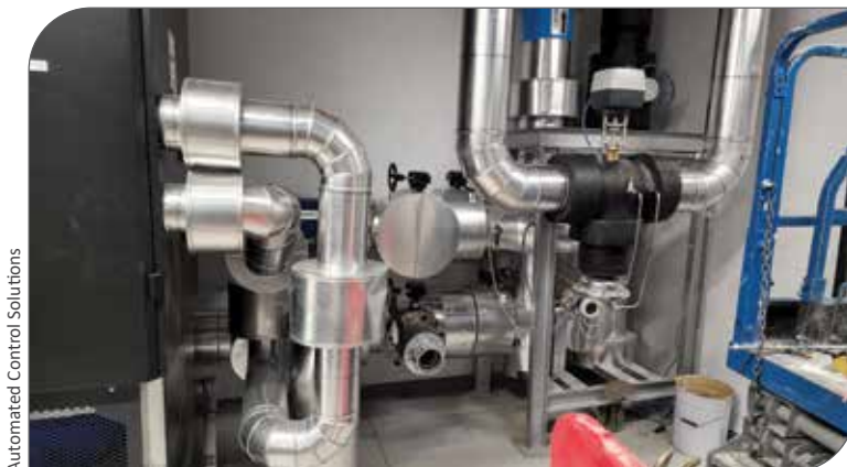
Danfoss ABQM DN150 installed at a local data centre.
