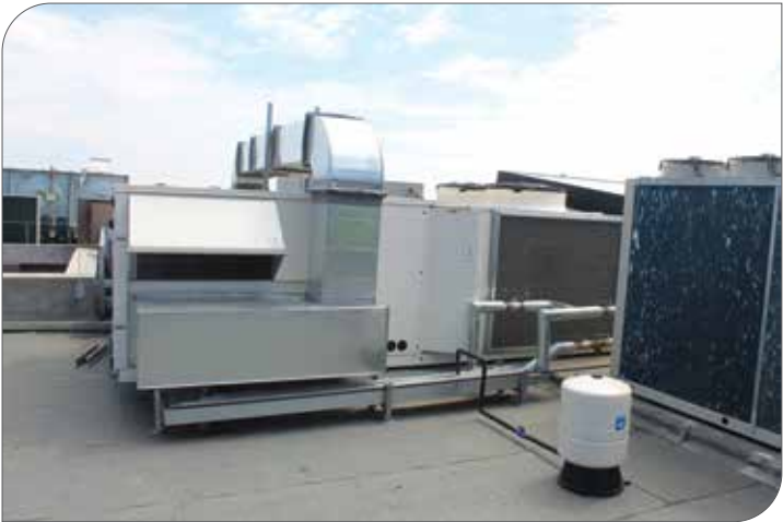
Roof-top package unit for tempering fresh air.
