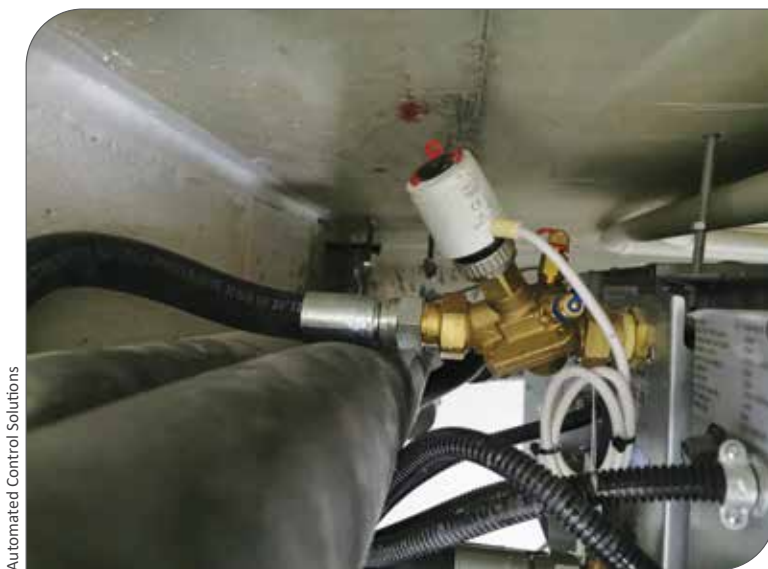
Danfoss ABQM FCU Valve and actuator installed in very tight space.
