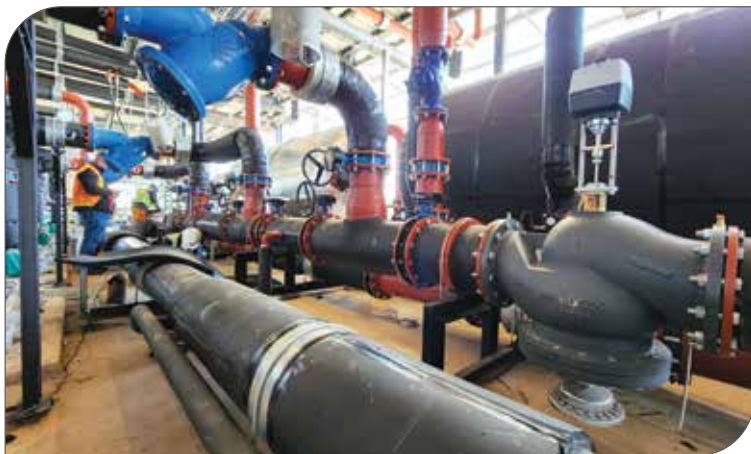
Danfoss ABQM DN250 at a local data centre.
