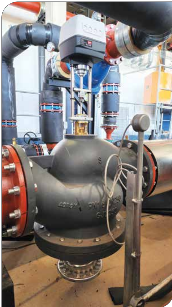
A DN250 Danfoss AB-QM PICV valve and actuator – one of six installed at a local data centre.
